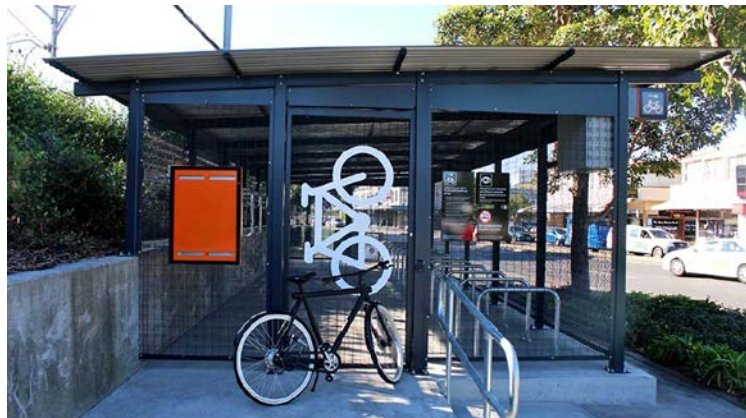
A bike storage rack at Caringbah Station (NSW) that will form the basis of the future mobility shed (Source: St George & Sutherland Shire Leader)
