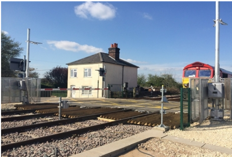
MCB-OD Level Crossing Technology [1]
