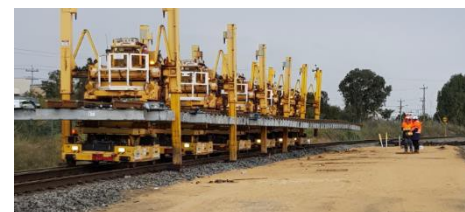
Figure 3 - Turnout moved into place by PEMs & LEMs
