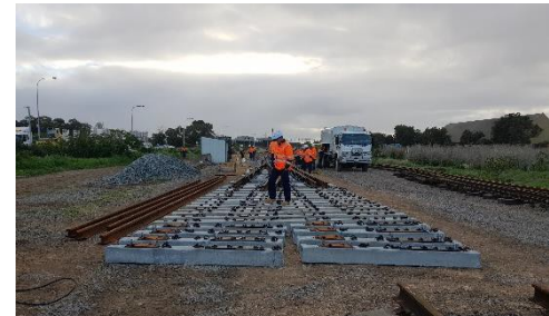
Figure 1 - Turnout built in-situ
