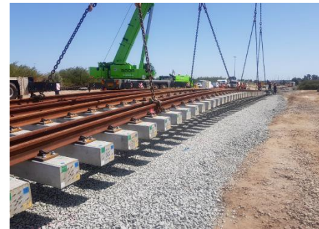
Figure 2 - Turnout installation with cranes
