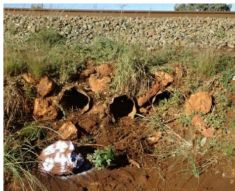
Figure 1 - Small Diameter Rail Culvert
