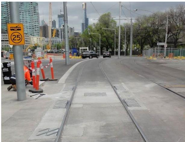
Noise reduction results for frequencies associated with tram squeals during pre-mitigation (i.e. non-TOR) FM noise monitoring (3150 and 5000Hz) have been reduced by 11-18.5dB, representing an approximate 50% reduction in subjectively perceived noise loudness existing prior to TOR incorporation. In addition, feedback received from area residents has been mostly positive.
