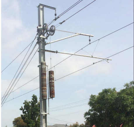
Figure 1 - Weight Wheel Tensioner
