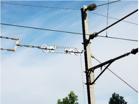
Figure 2 - Pulley Wheel Tensioner
