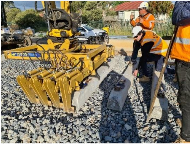
Photo 1: Sleepers being laid with labourers close by
