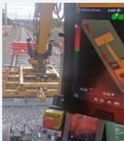
Photo 2: Sleepers being laid with machine control
