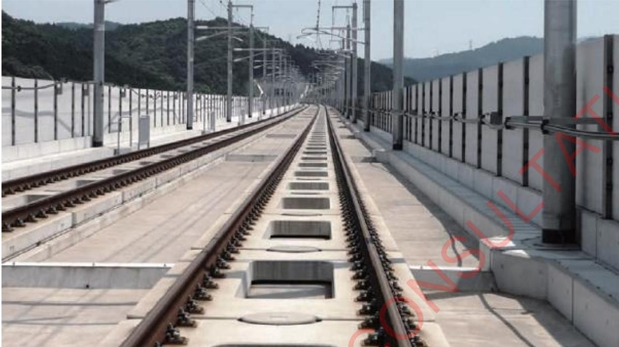
*Appendix Figure A.4-1 Example of precast slab type ballastless track system*
