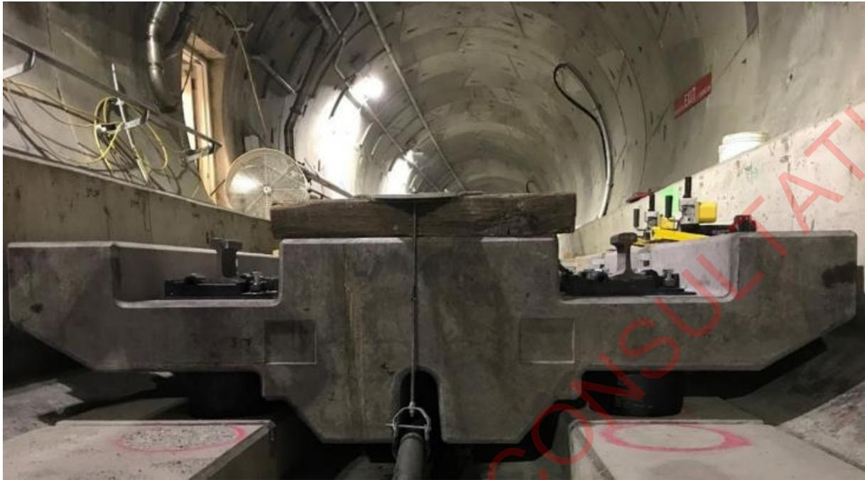
*Appendix Figure A.7-1 Example of typical floating slab track system*
