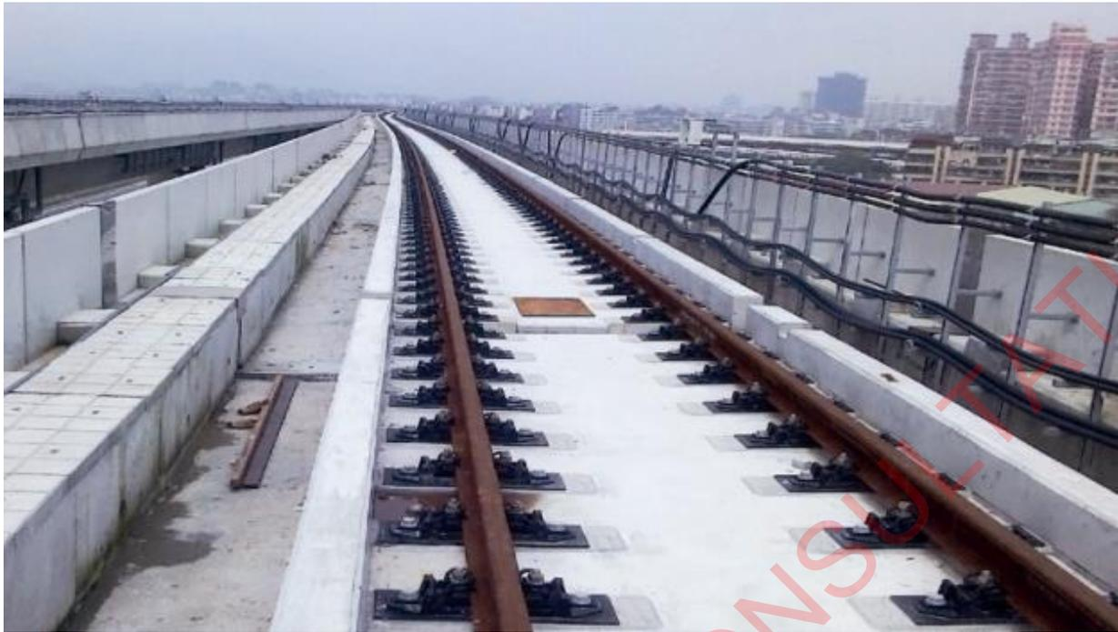
*Appendix Figure A.5-1 Example of in-situ monolithic slab system*
