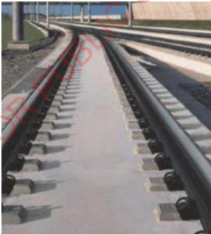
*Appendix Figure A.2-1 Example of embedded sleeper type ballastless track system*
