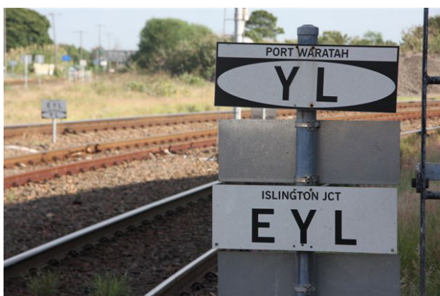
Example track warrant intermediate board used in NSW - a notice board provided between stations or sidings to identify a location that may be used to designate a limit for a track warrant.
