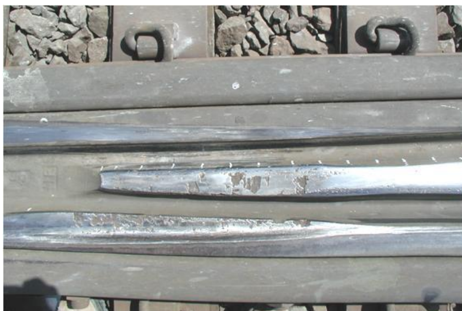
Figure A7: Heavy deformation at crossing nose and wing rail
