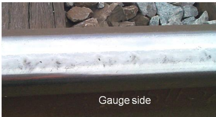
Figure A5: RCF on the gauge corner of the outer rail in a curve
