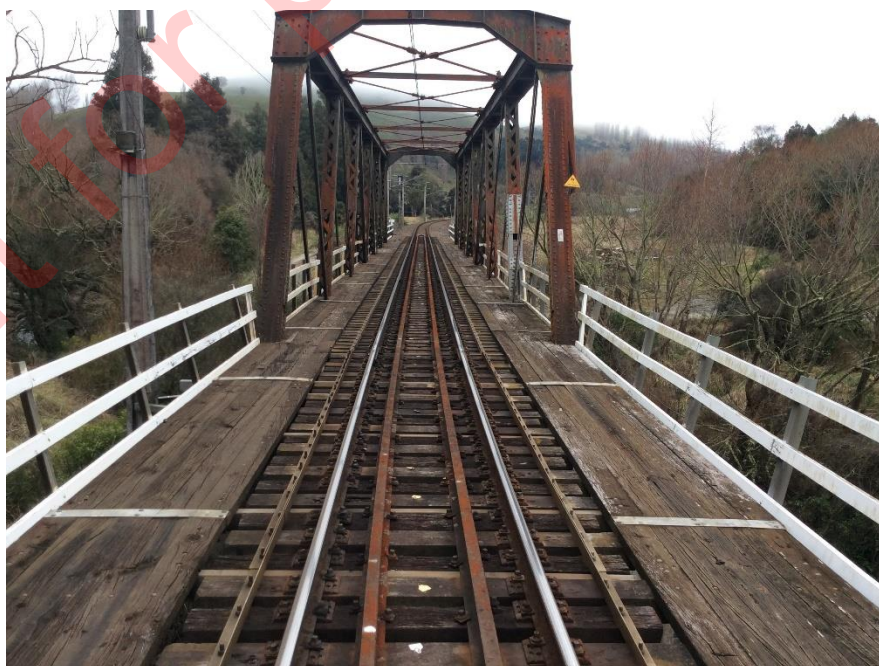
Figure A-2: Example of through truss design with truss elements above deck height
