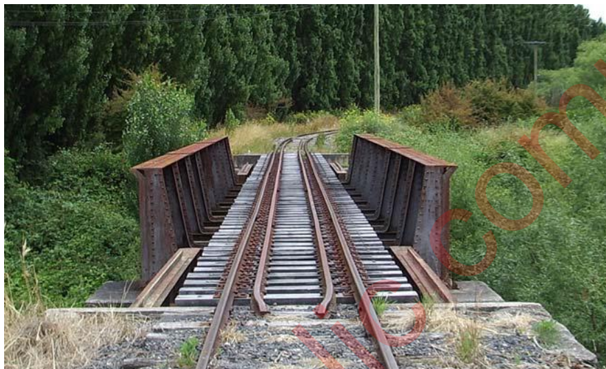
Figure A-1 Example of through girder design with structural girders above deck height
