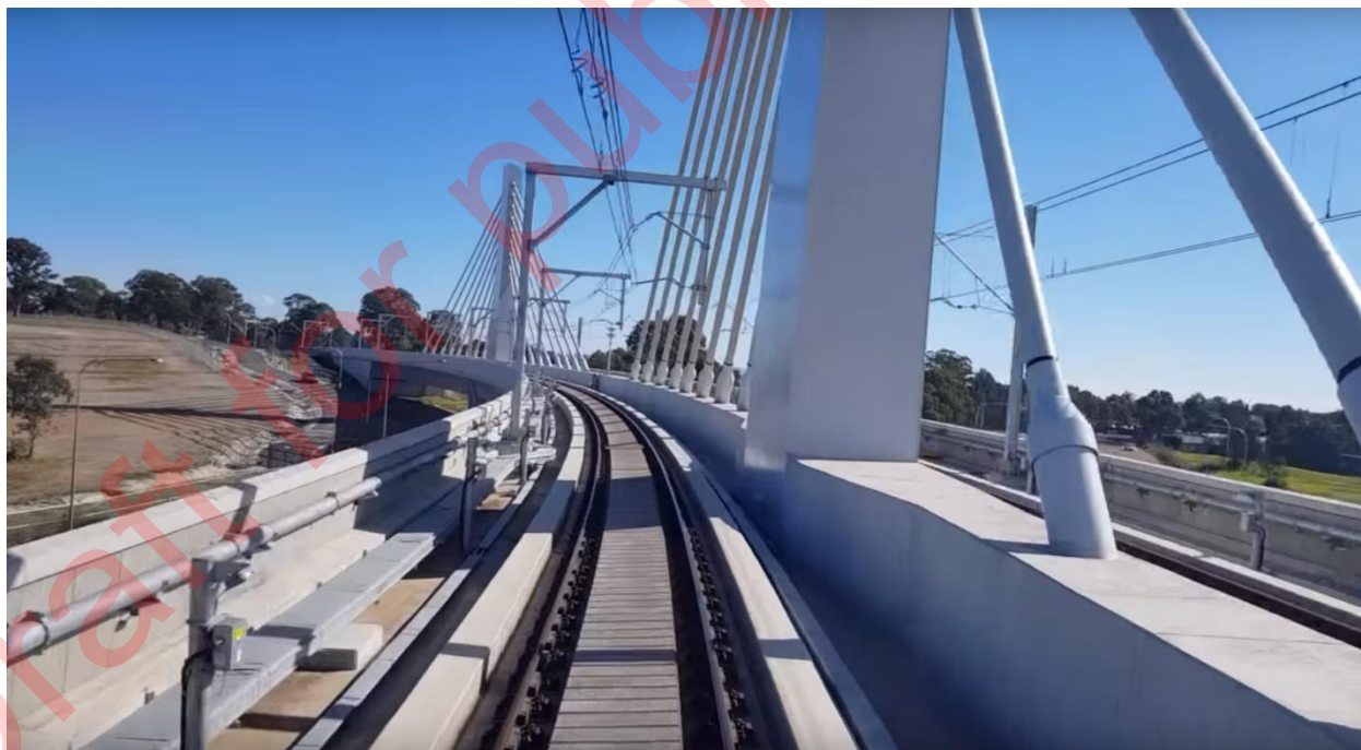
Figure B-3 Example of derailment kerb, impact protection barrier and deflection wall
