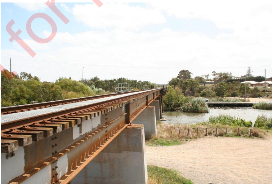
Figure A-4.: Example of transom top bridge. Structural members are below deck
