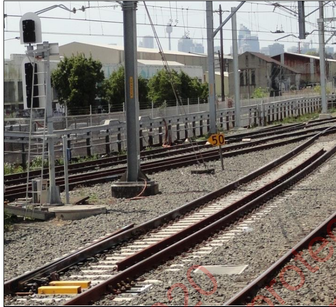
D3:2 - Catch point – single blade with an internal guide rail
