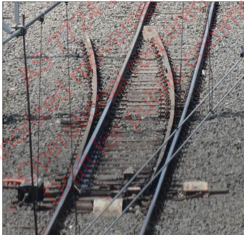
D2:1 - Catch point – double blade with an internal guide rail
