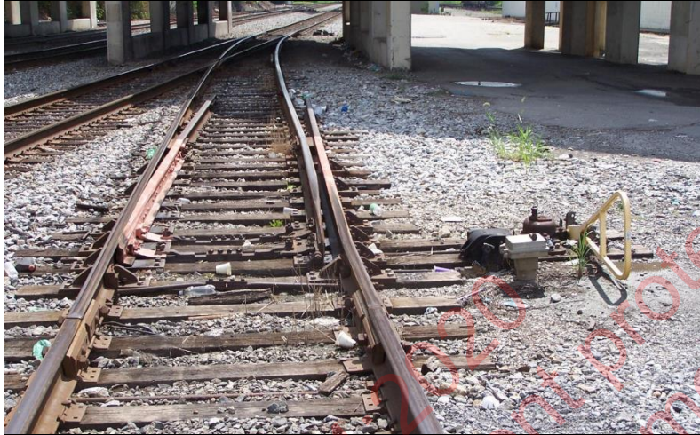
G1:1 Poorly located catch point
