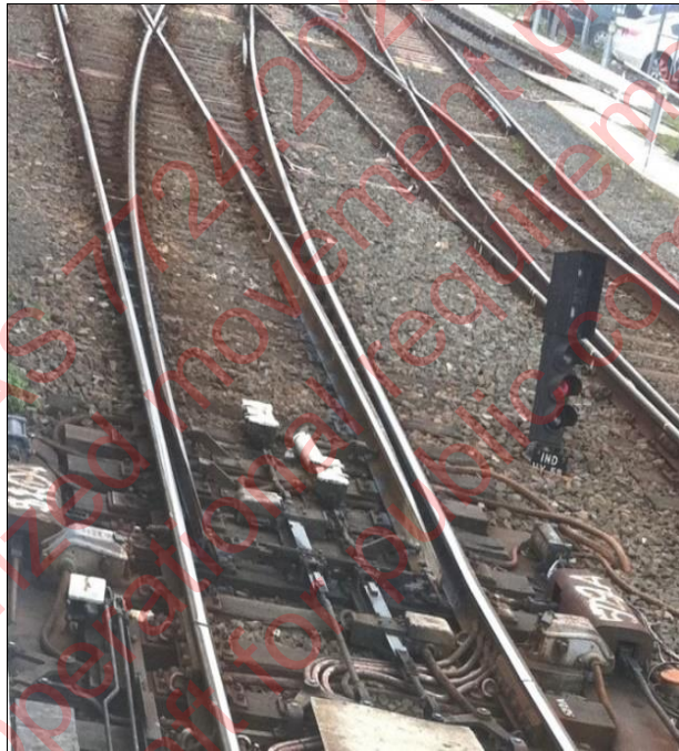
D5:1 - Catch point – two individual blades or independent switches
