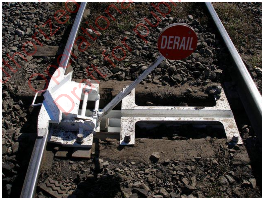
C1:2 - Bi-directional derailer with flag indicator
