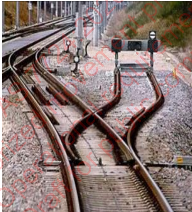
D4:1 - Catch point – double blade with run-off
