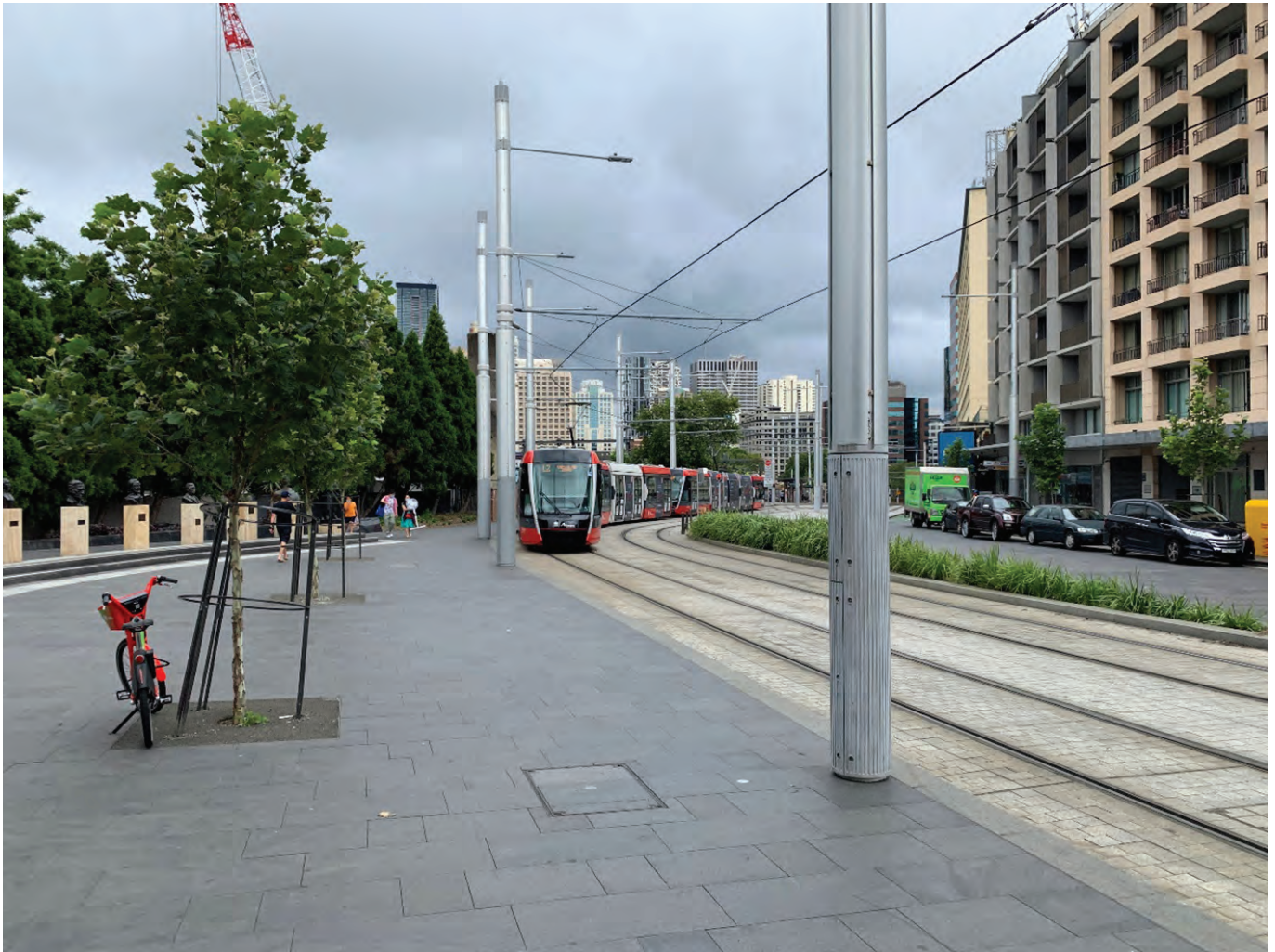
Figure 21 Light rail systems often feature rails embedded in the road. Grease on these rails can be hazardous to pedestrians, cyclists and motorised road traffic.
