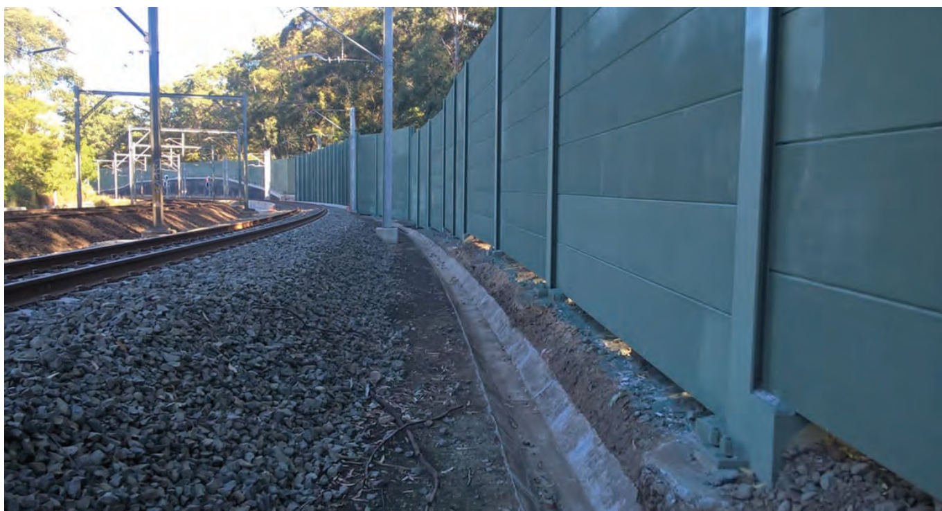
Figure 27 Noise barriers on the Epping to Thornleigh Third Track project to mitigate wheel squeal, locomotive and general rail noise (89)
