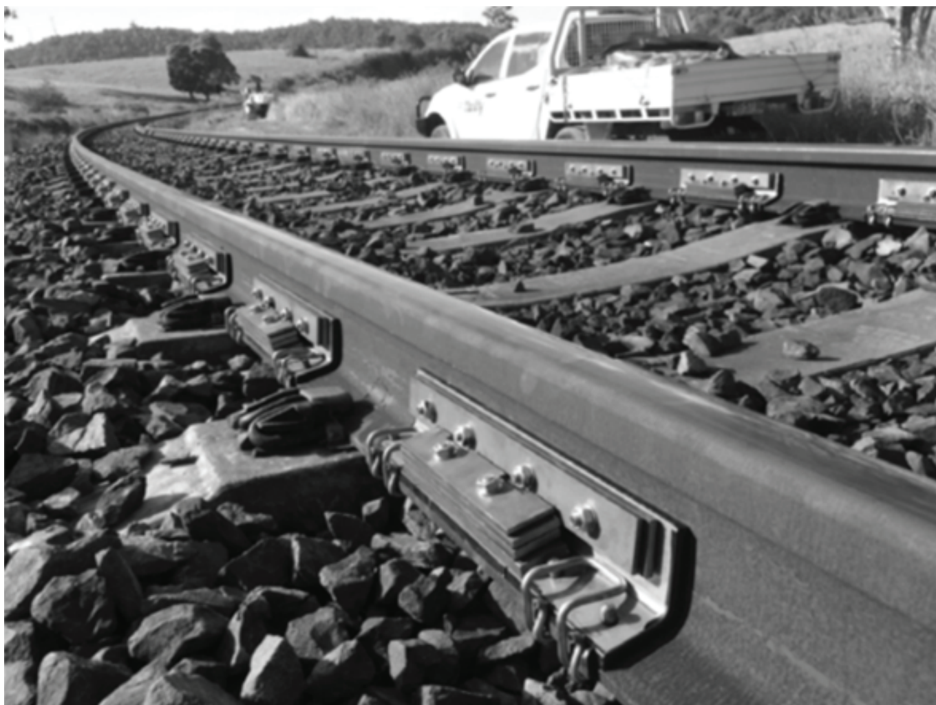
Figure 26 In a NSW trial, rail dampers reduced wheel squeal noise by a modest amount (27)
