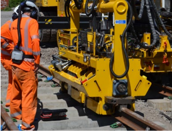
Induction Welder on Track (Source: Mirage Ltd)
