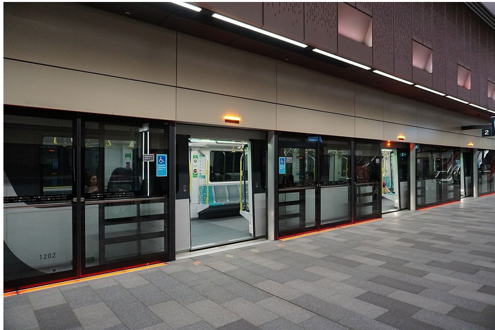
Figure 1: Platform Screen Doors at Castle Hill Station on the Sydney Metro (Source: https://commons.wikimedia.org/wiki/File:CastleHillMetroStation.jpg )
