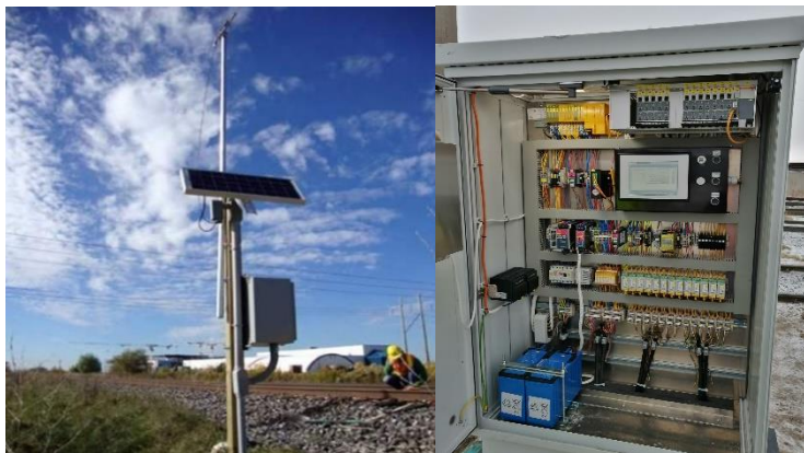
Figure 2 Pole mount wireless axle counters wayside junction box with solar
