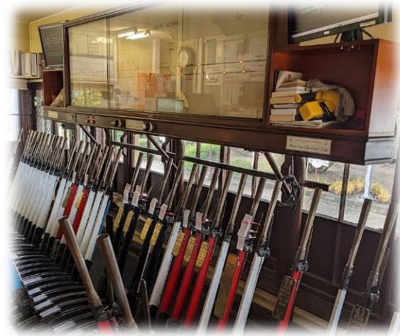
Figure 3 Mechanical Interlockings - final days before decommissioning
