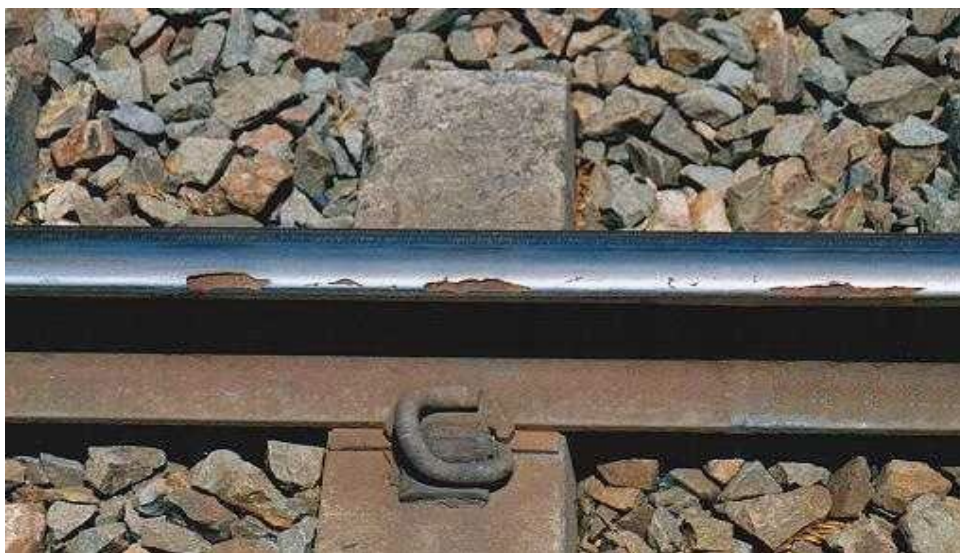
Appendix Figure D.19 Head shelling
