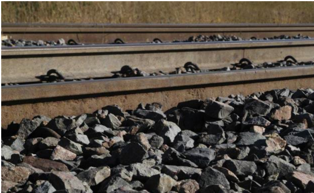
Appendix Figure D.13 Corroded rail
