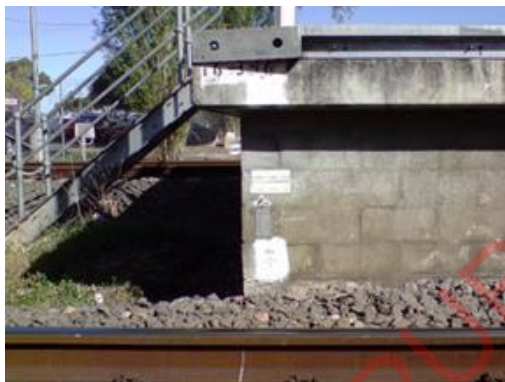
Appendix Figure E-5 Brass bar TCM in platform
