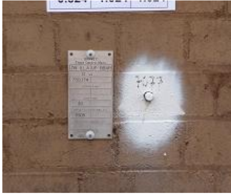
Appendix Figure E-1 Brass bar and survey plaque
