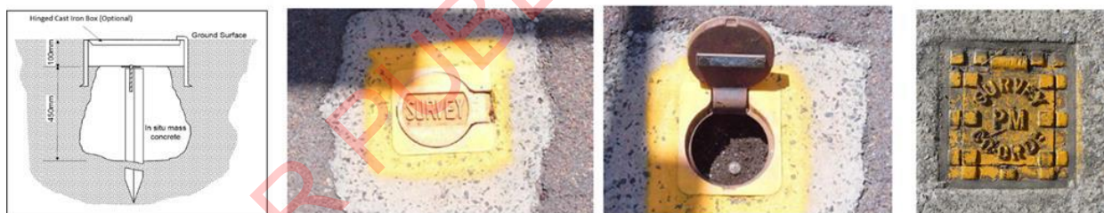
Appendix Figure D-3 Survey marks in cast iron cover boxes
